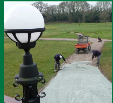
The final touches to the new paths by the terrace
